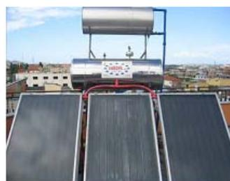
Figure 1. Photo of Solar Water Heating System No. 4 - Production of "EUROPA A.P.", Durres
